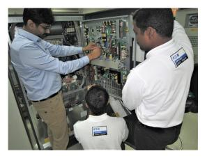
Major PM Visits will require that the UPS be put into "bypass" and isolated so the UPS can be safely inspected including its internal components. See UPS below.
