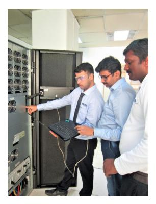
We will vacuum and/or blow out dust and debris, inspect air filters and replace as necessary. Close inspection of capacitors will occur with meter testing where deemed necessary. (Sencore LC53 capacitor-inductor meter) All cables and connections will be inspected and checked for tightness and re-torqued where necessary. Seating of components and control wiring is checked.
